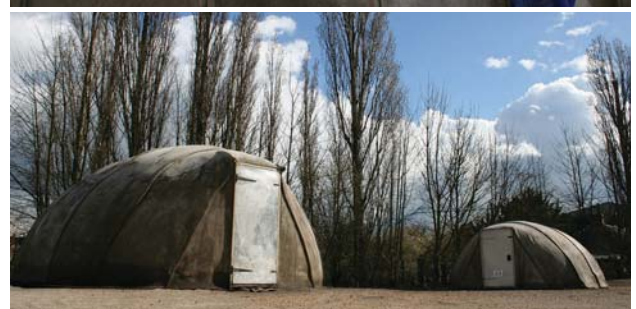
Delivery, inflation, hydration and setting for 54m 2 shelter.
