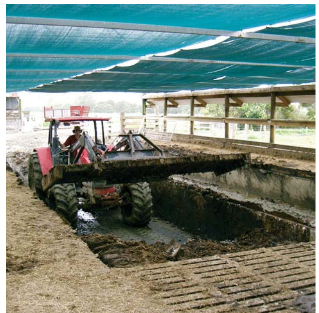
Concrete floor grates removed for effluent collection.
