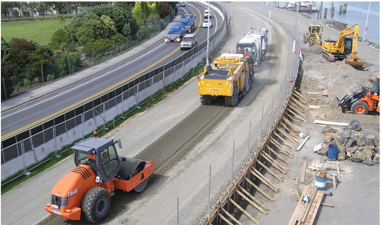
The latest in dustless cement stabilisation on Hewletts Rd
