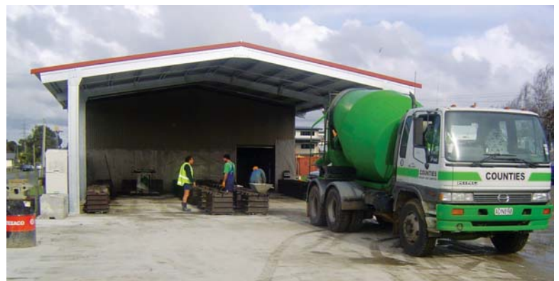
Interlocking block production using residual concrete.
