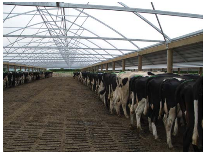
A Herdhome® shelter - prestressed concrete grated floor.
