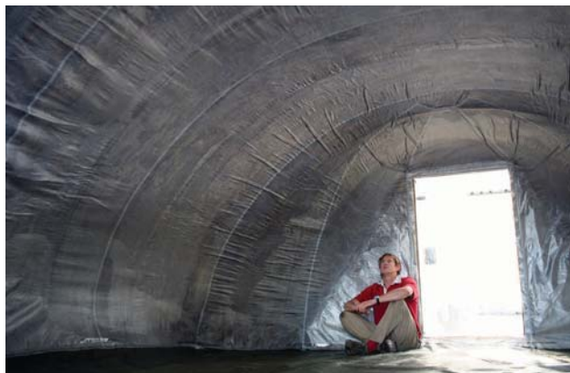
Interior of a concrete canvas shelter.
