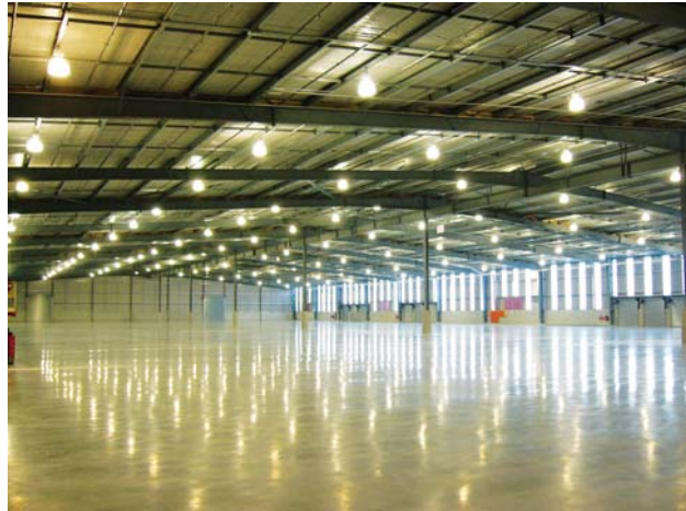
Fonterra storehouse - New Zealand's largest post-tensioned floor.
