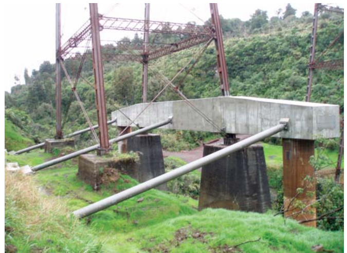
Makatote Viaduct - Pier 7 concrete crossbeam and steel struts.
