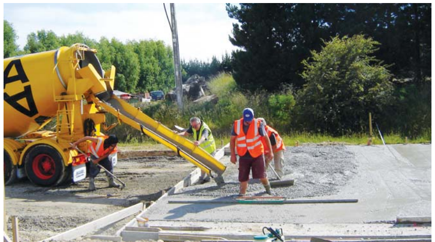
Concrete Pavement pour - Setters Line, Palmerston North.
