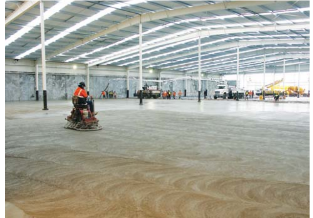
Fonterra storehouse - post-tensioned floor finished using eight rideon paver trowels.
