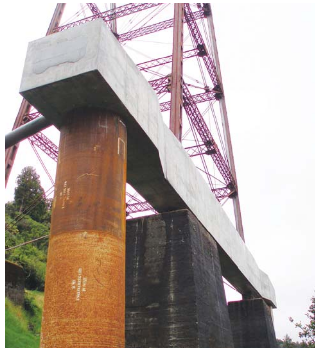
Pier 7 strategically shaped crossbeam, reduced concrete volume and load requirements.
